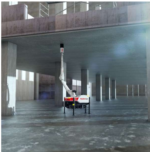
Figure 1 BauBot Ceiling Installation
