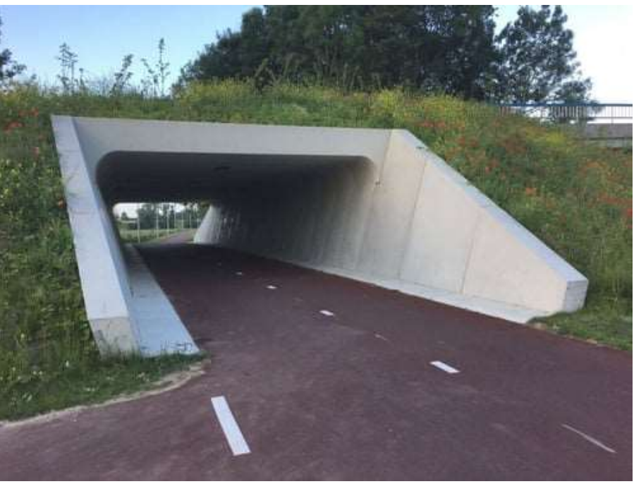
In situ poured concrete
