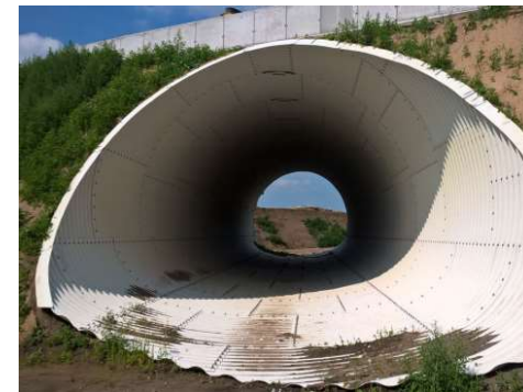
ViaCon – bicycle tunnel Rieme (BE)
