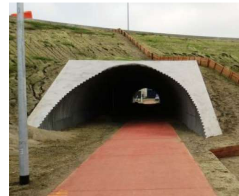
Altena – bicycle tunnel Beveren (BE)
